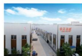
湖北铁正立加厂区 Hubei Tiezheng Vertical Machining Plant
